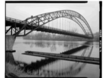
Bellos Falls Arch Bridge
