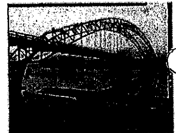
Bellos Falls Arch Bridge
